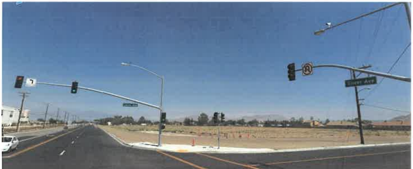
Project site looking Southeast from the intersection of Slover Avenue and Laurel Avenue.
