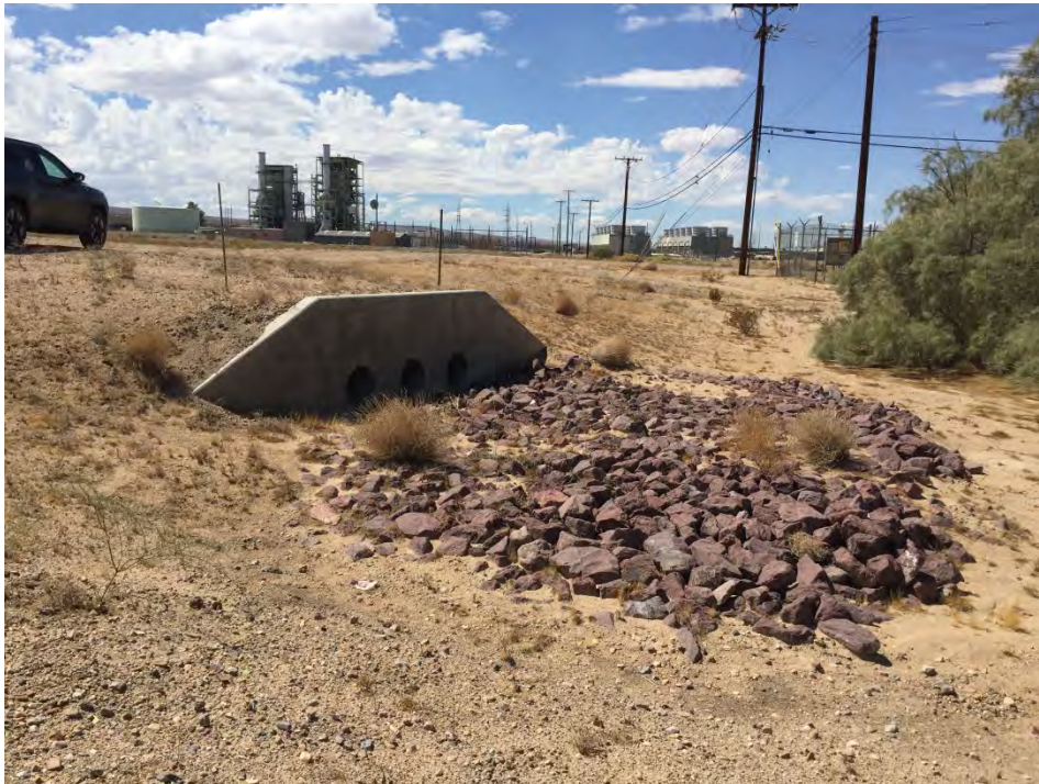
Photograph 8. Culvert intended to convey runoff from ponds associated with the decommissioned energy plant under a dirt access road and into an isolated basin. View looking southwest.
