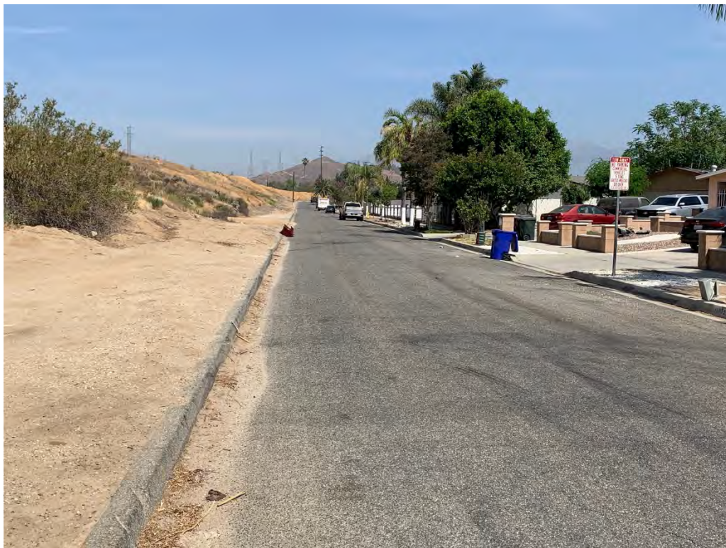
Photograph 4: Storm drain alignment in existing road.
