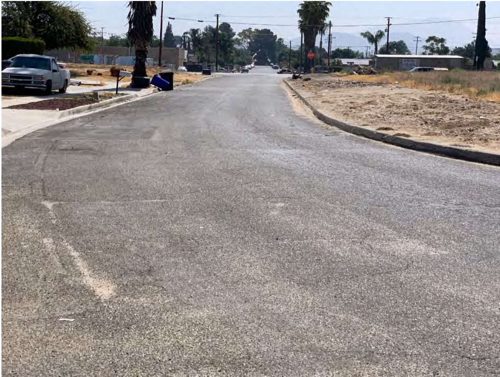
Photograph 5: Storm drain alignment within existing road.
