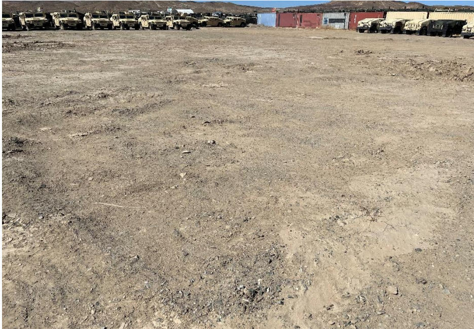
Project overview from near northeast corner, view to southwest.
