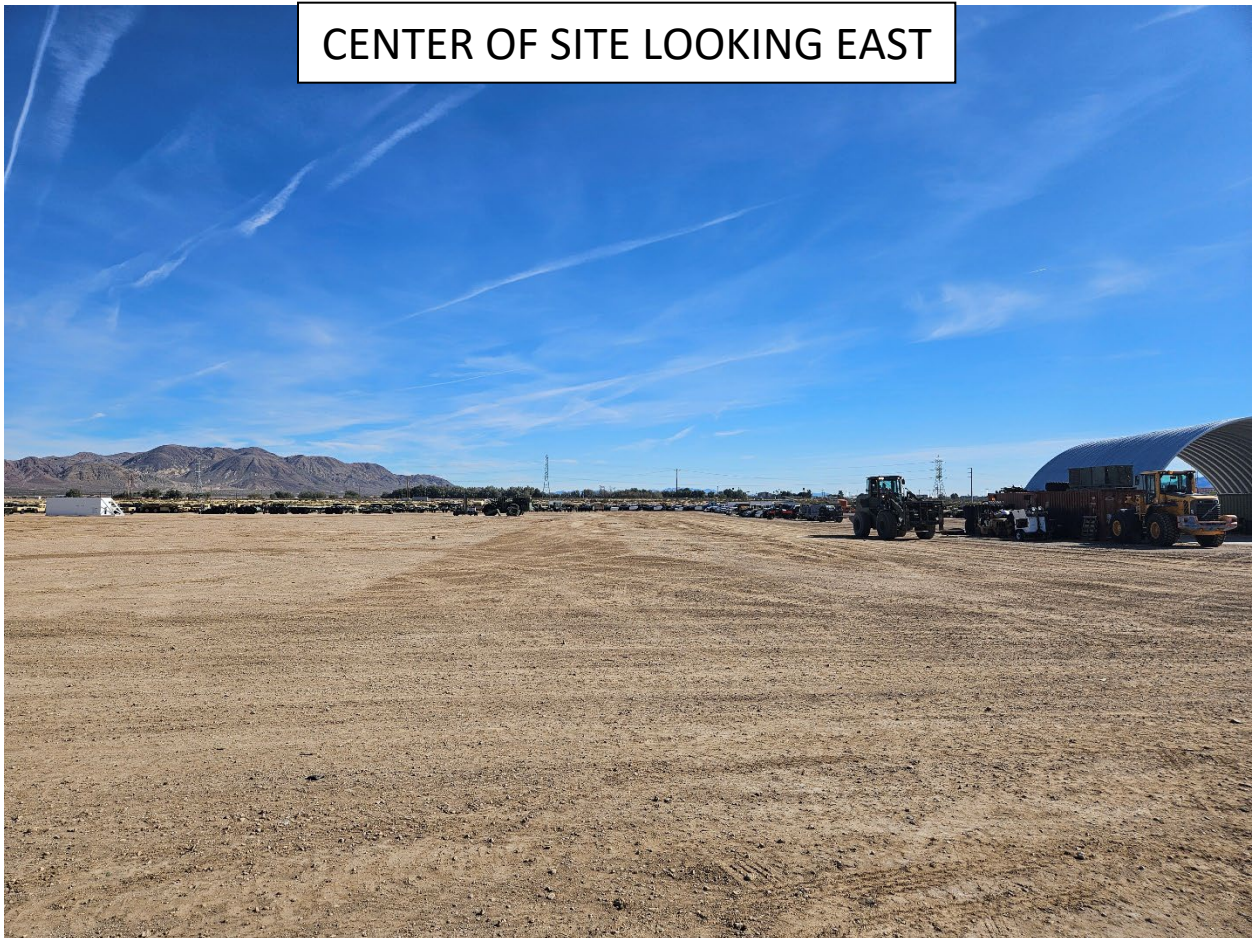
FIGURE 3: PHOTOGRAPHS OF SITE
