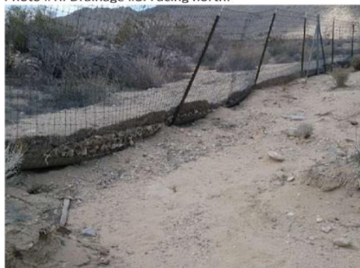
Photo #18. Drainage # 5. Deposition along perimeter fence.
