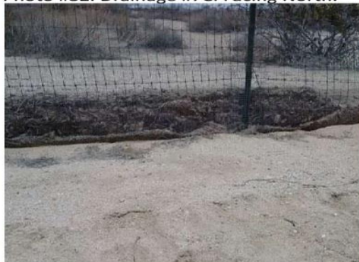
Photo #31. Drainage #8A. Deposition at perimeter fence.
