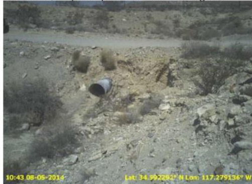
Photo #4. Quarry Rd. Upstream of Site. 3 ft wide culvert. Drainage #3.
