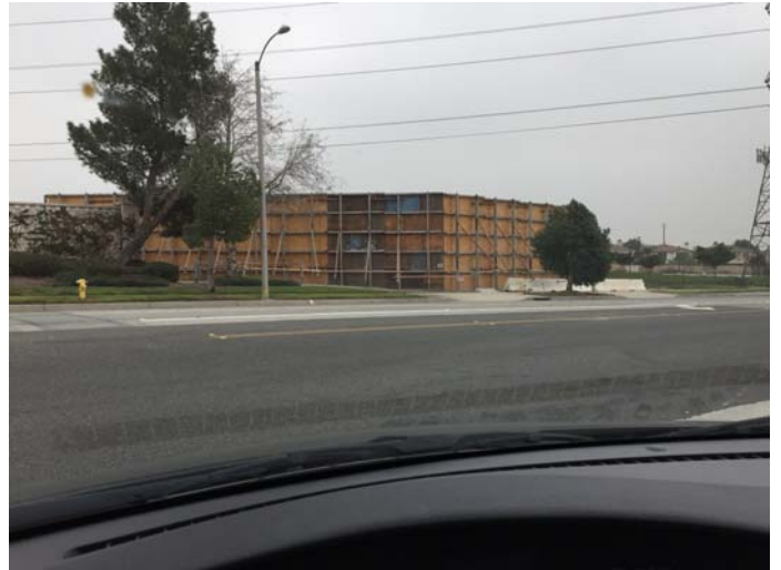
K-Rail Plywood & Acoustic Material
