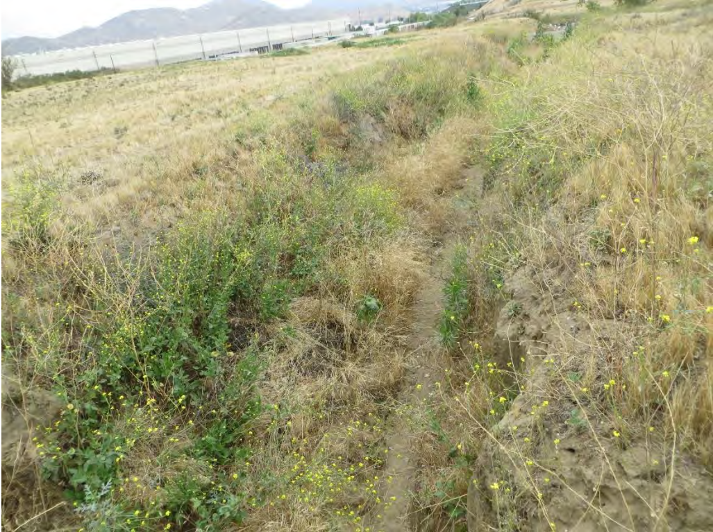
Photograph 3: Facing east along Drainage A.
