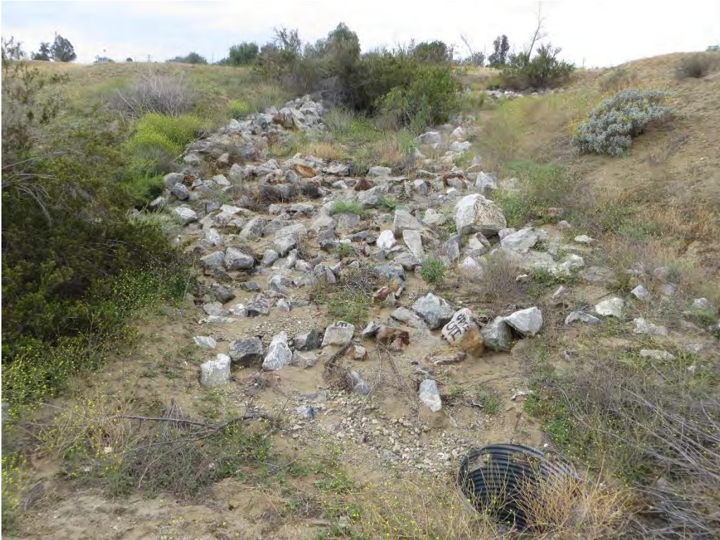
Photograph 6: Facing southwest at the detention basin and inlet to downstream waters.
