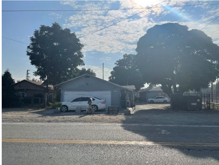
Photograph 8: 11635 East End Avenue, west façade, facing east Photo taken by Tetra Tech, 9/14/22.
