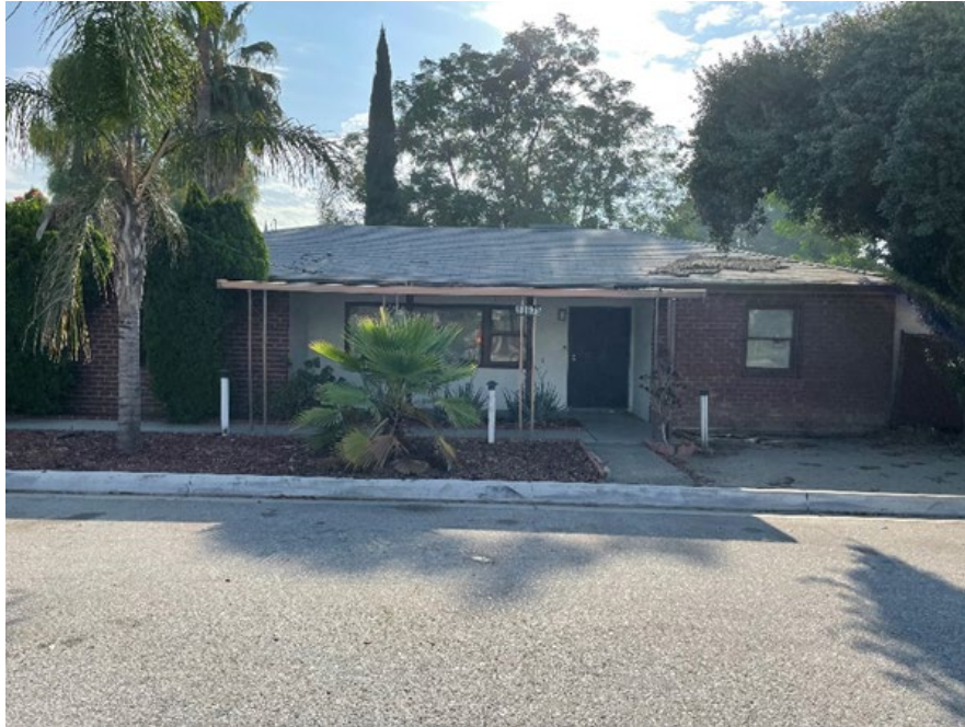
Photograph 4: 11675 East End Avenue, west facade
