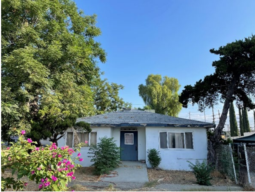
Photograph 2: 3730 Francis Avenue, main facade, facing north
