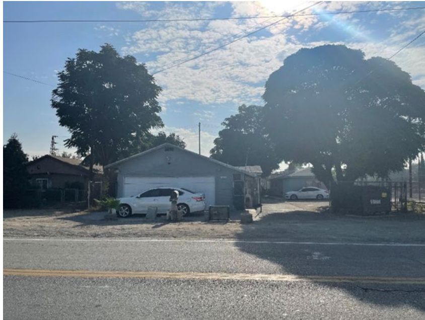
Photograph 8: 11635 East End Avenue, west facade
