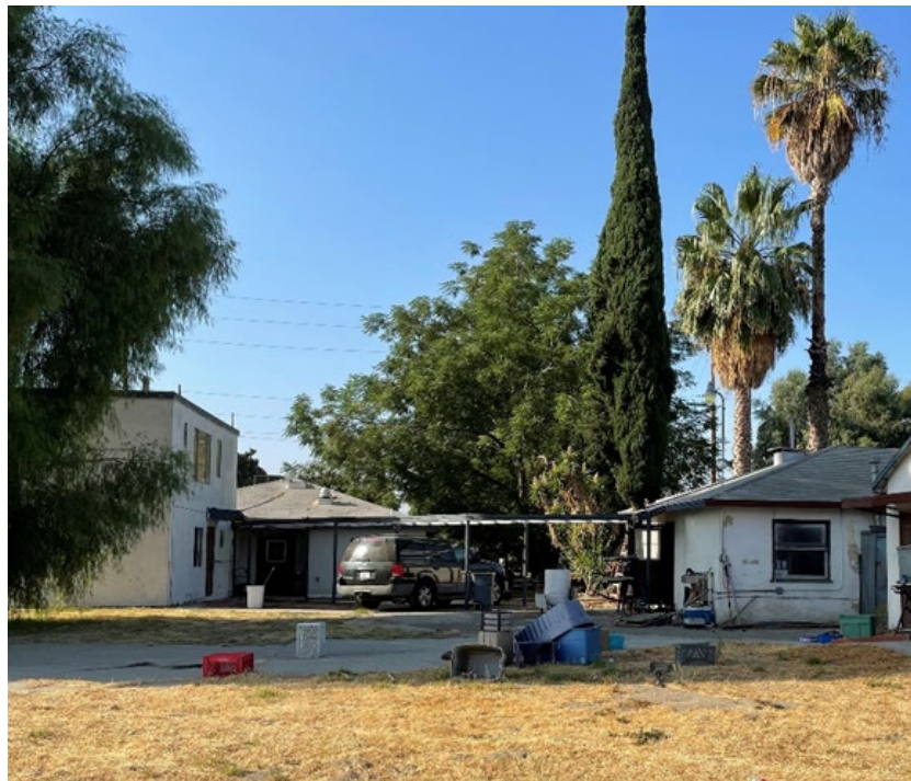
Photograph 7: 11641 East End Avenue, north facade
