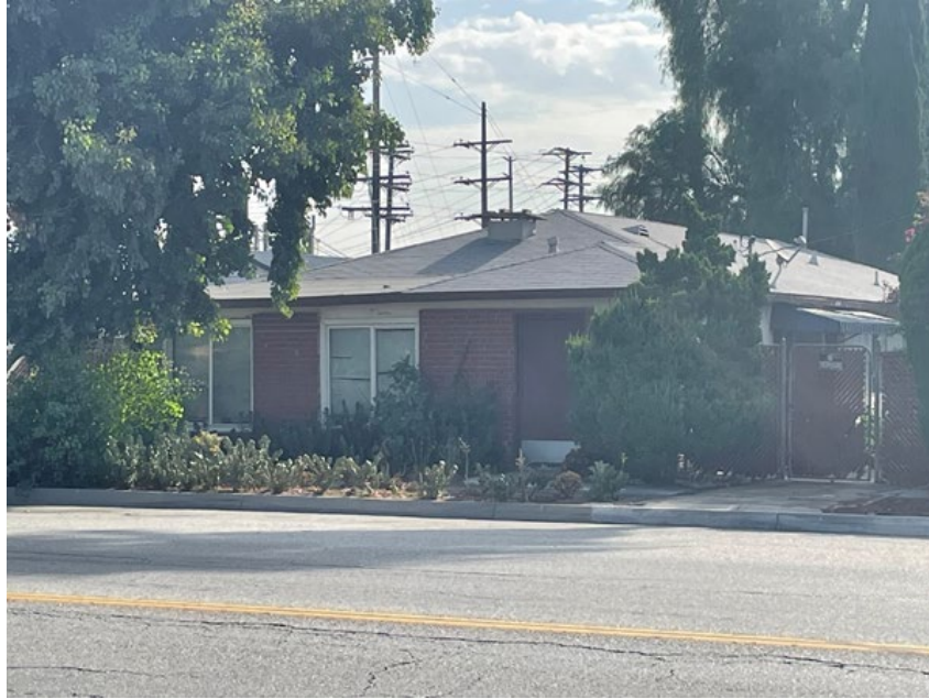
Photograph 6: 11641 East End Avenue, west facade
