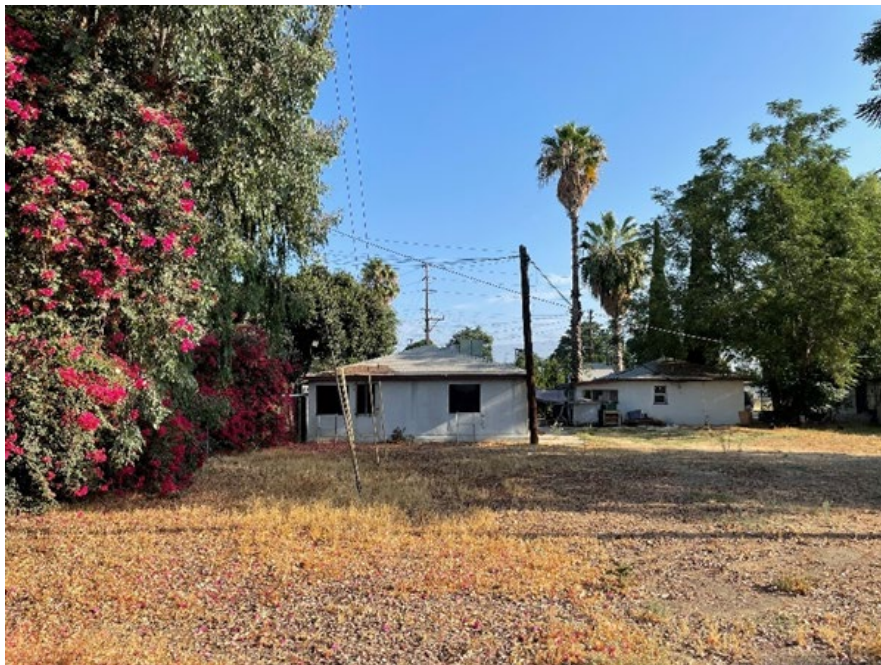
Photograph 5: 11675 East End Avenue, south facade
