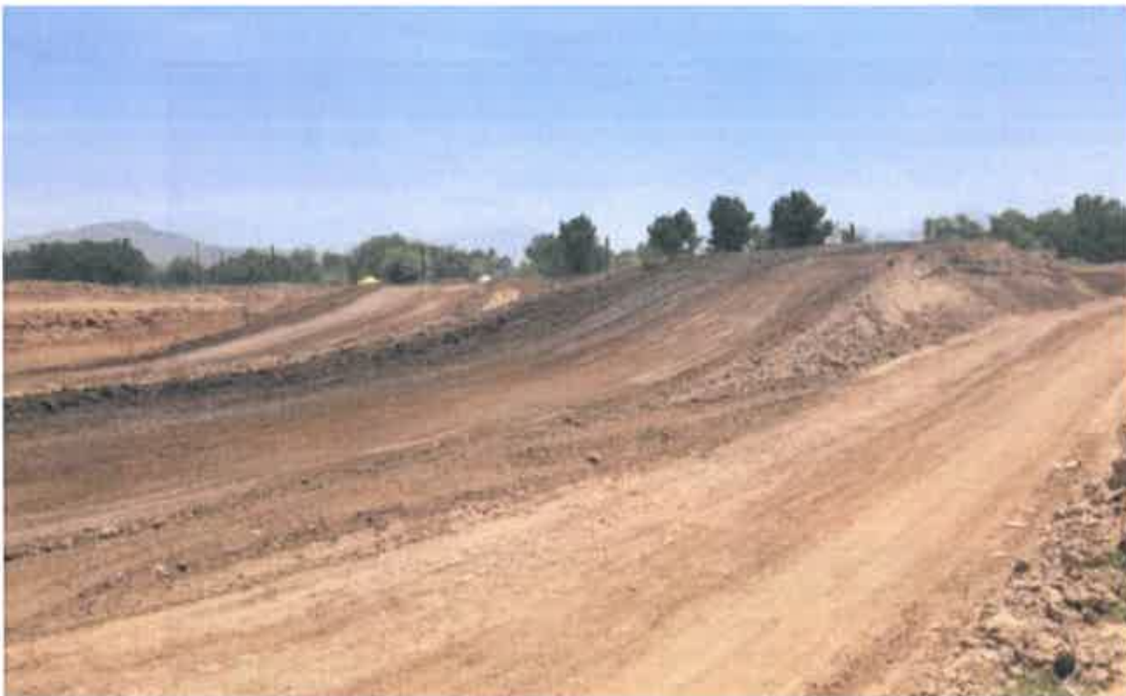
View towards south
