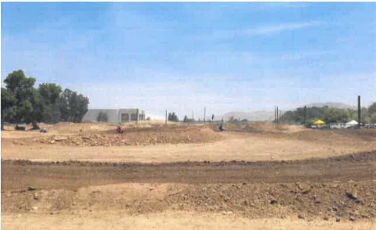
View towards northwest
