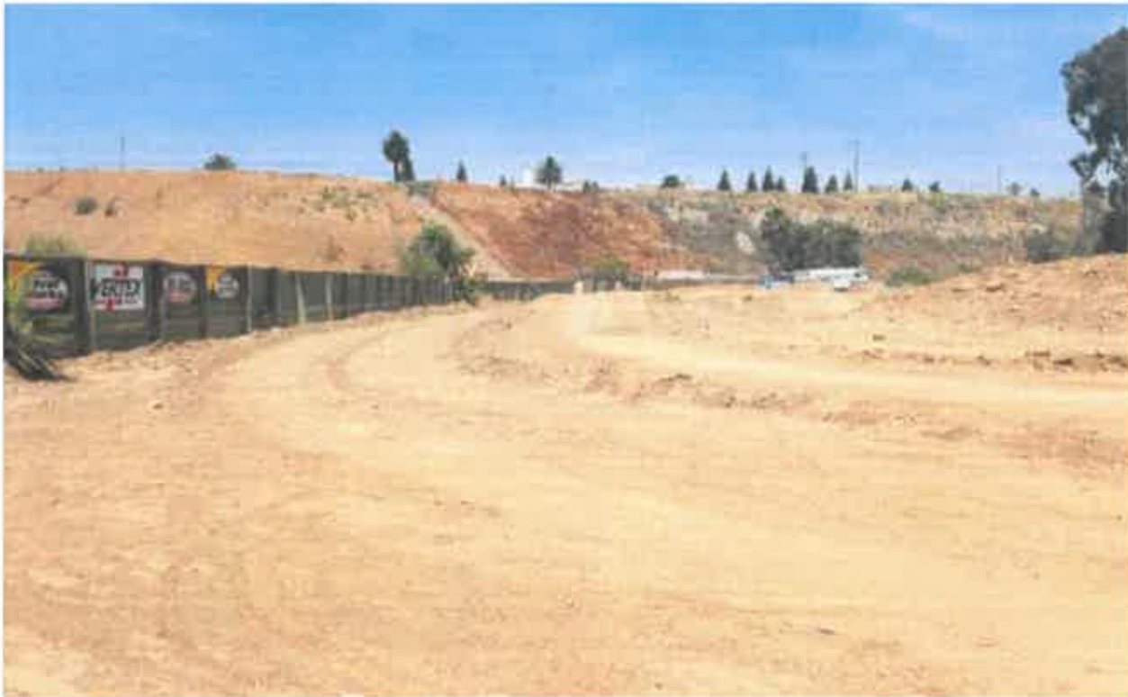
View towards northeast
