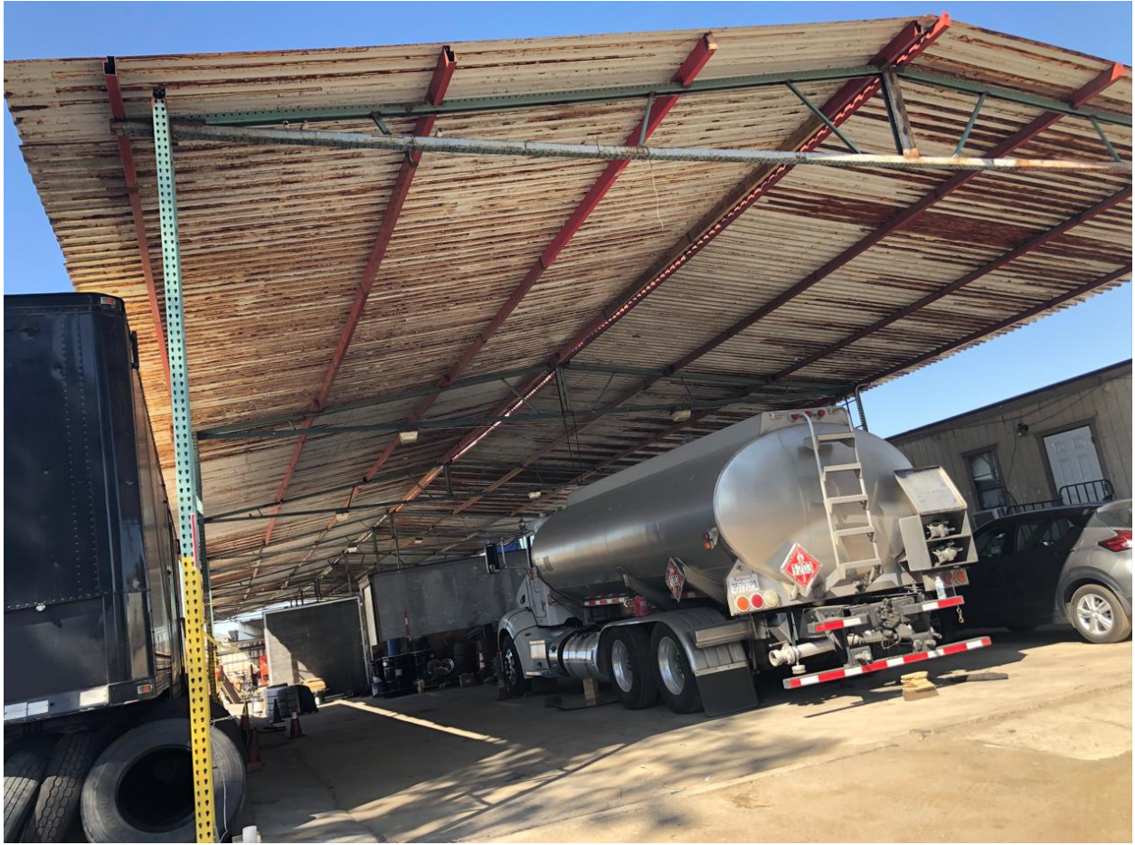
Existing metal canopy structure.
