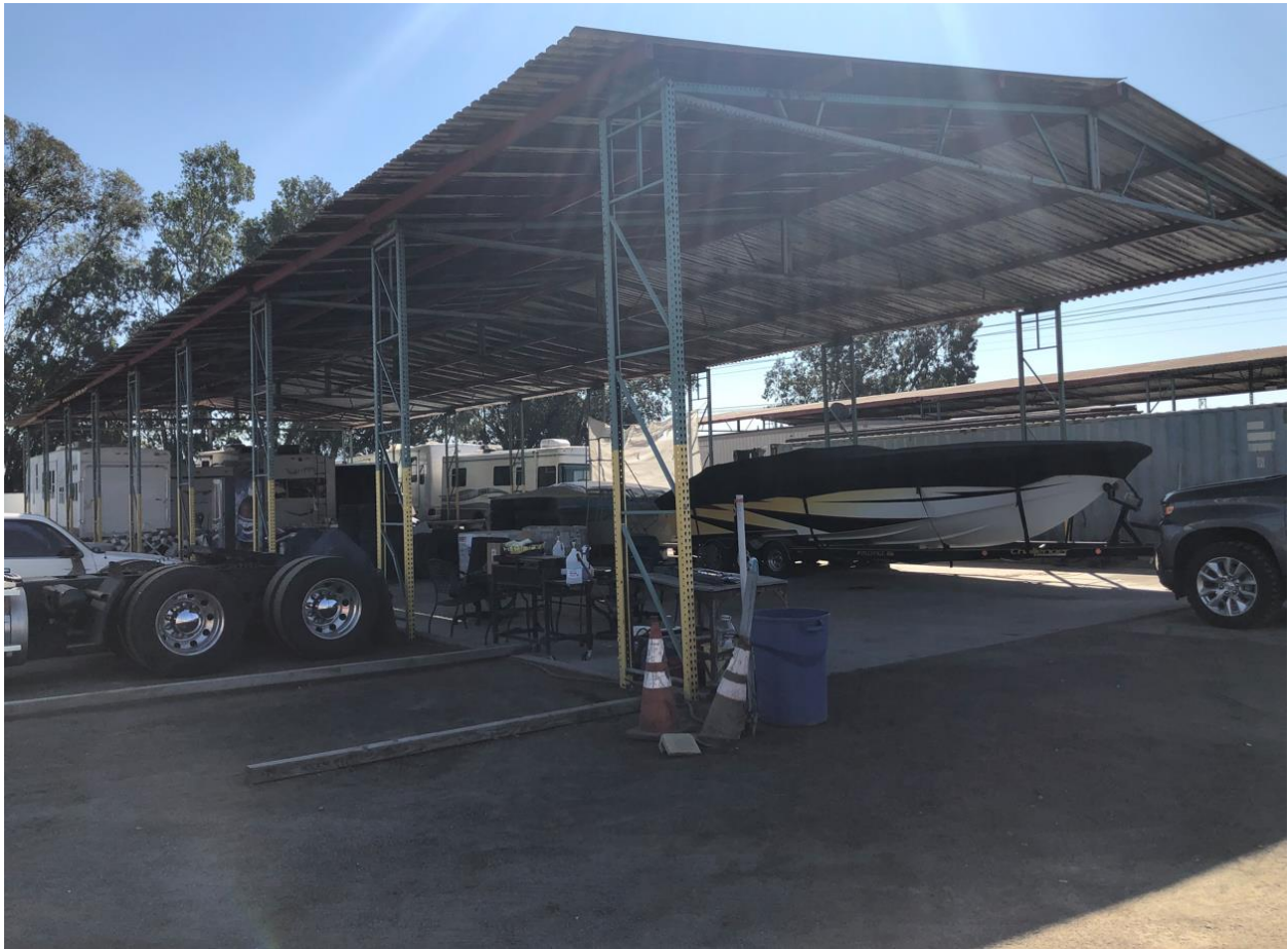
Second existing metal canopy structure.
