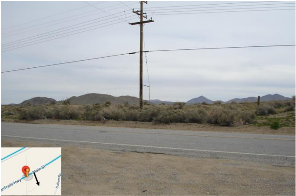
Pic I: Southeast from Corral Road towards vacant land and regional powerpole connection.
