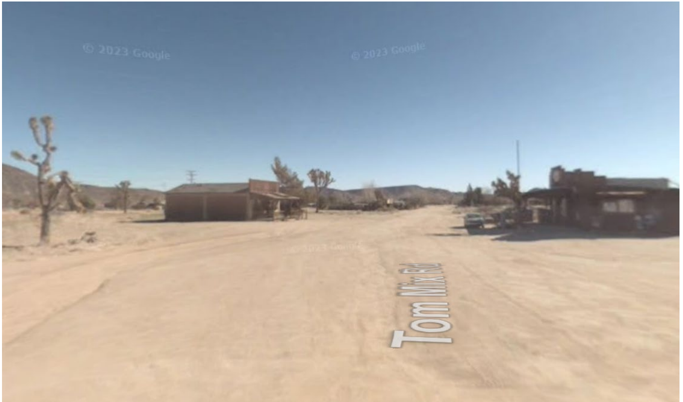
Photographs 5: Looking east from corner of Tom Mix Road and Mane Street with US Post Office south of the existing vacant building.
