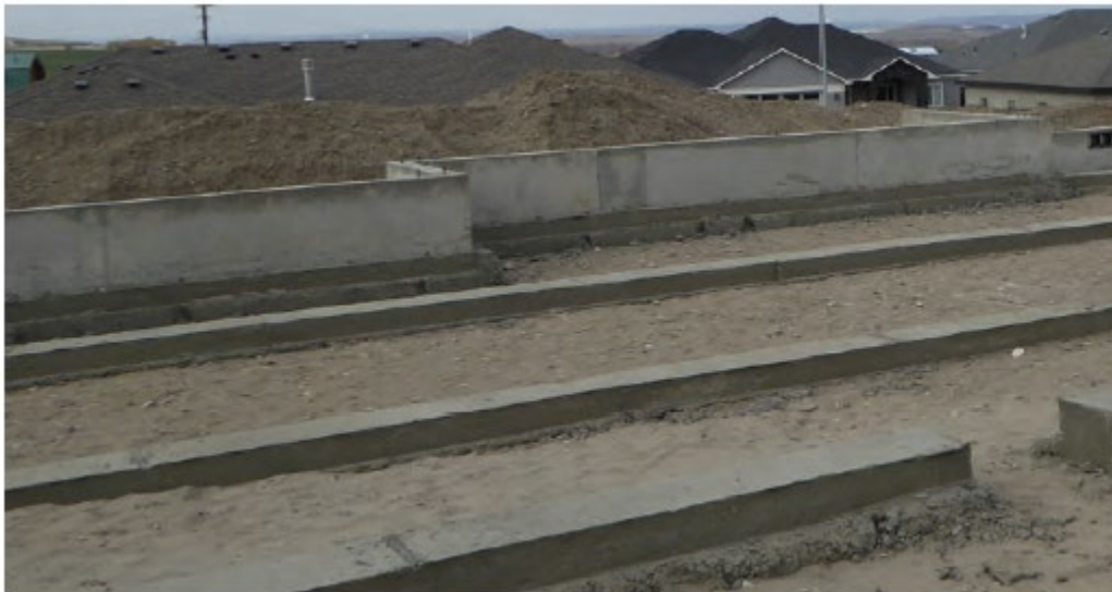
Stem wall and interior footings.
