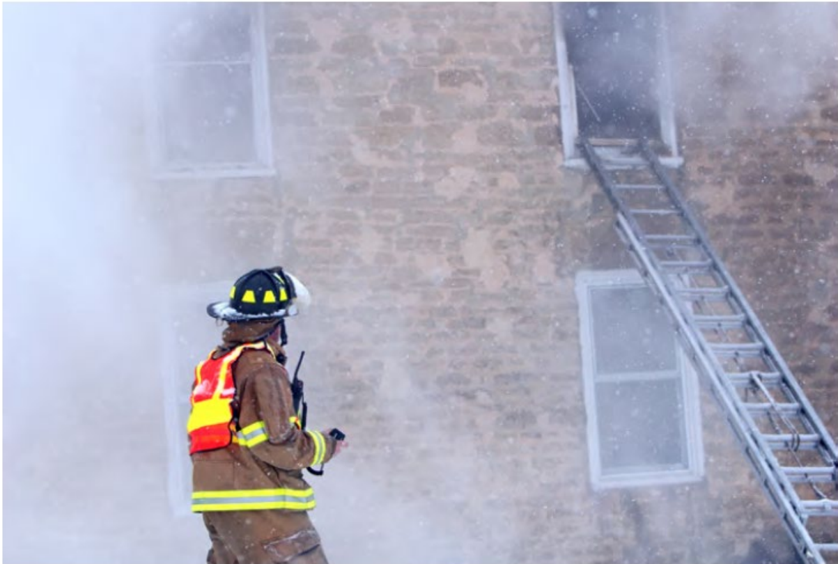
An emergency escape and rescue opening in use during a fire.
