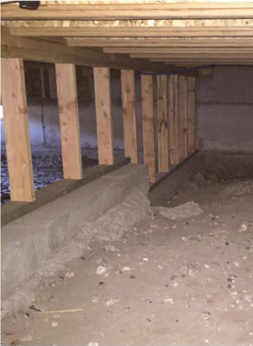
Interior cripple wall.
