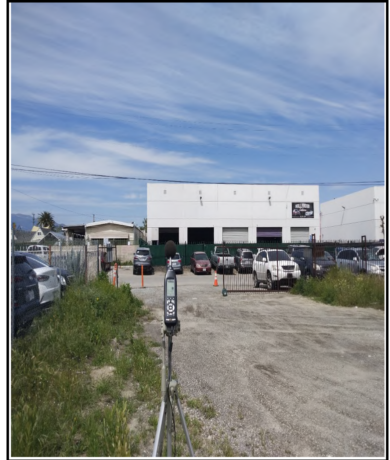
NM3 looking N from western edge of site across Taylor Ave towards commercial building, 17763 Valley Blvd, Bloomington.
