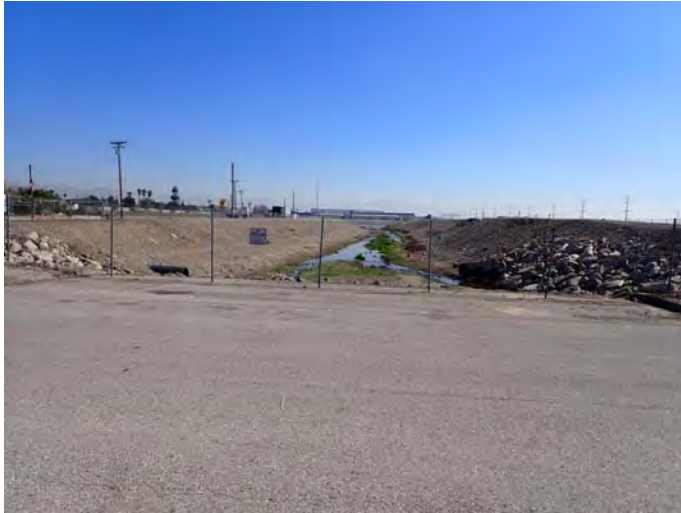
13) View of the site drainage swale along the south side of Whittram Avenue.
