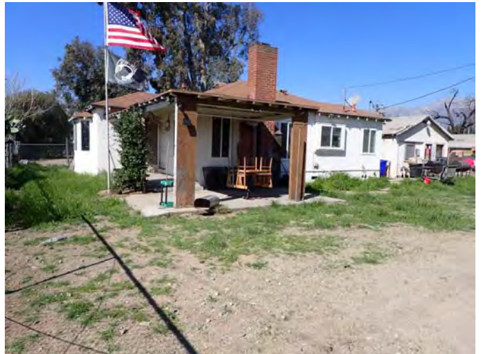
12) View of the exterior at the main house, 13932 Whittram Ave.
