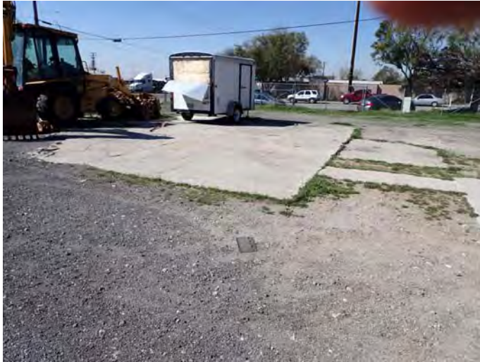
5) View of the former residence slab at 8733 Calabash Ave.
