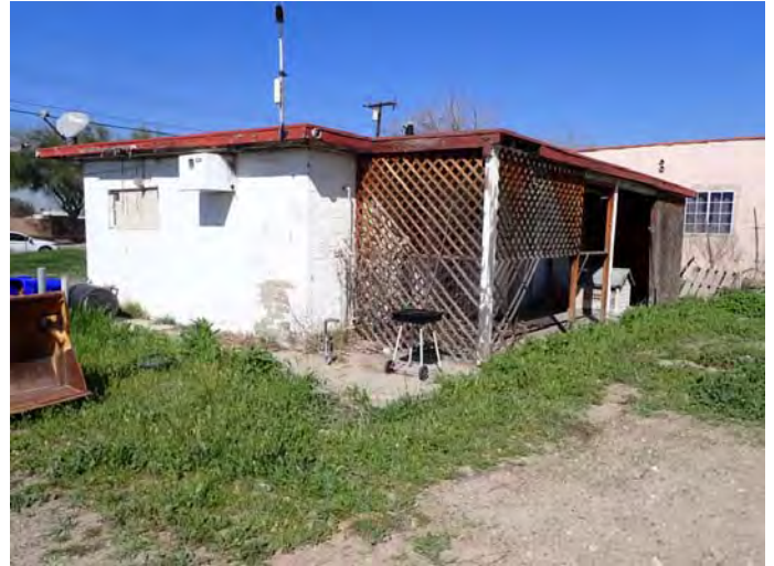
6) View of the CMU residence at 8721 Calabash Ave.
