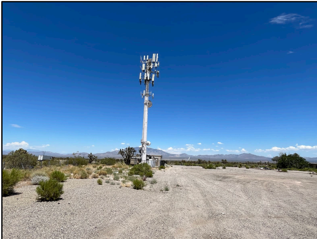
Plate 3.2–6: Overview of cell tower area and associated infrastructure, facing northeast.
