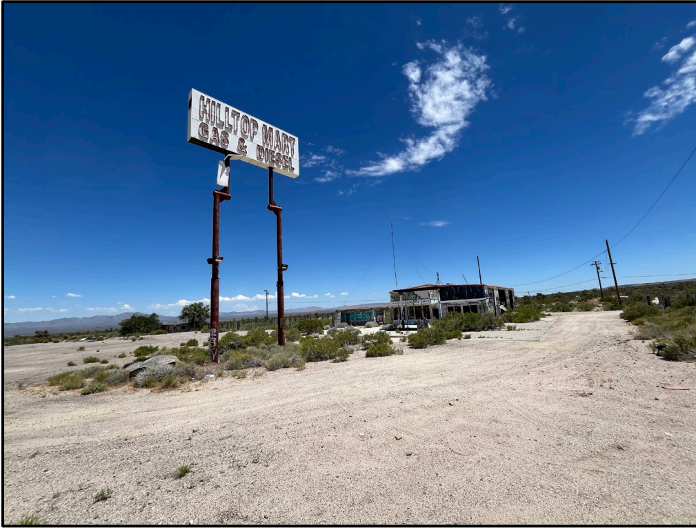
Plate 3.2–3: Overview of the subject property and former gas and service station, facing south.
