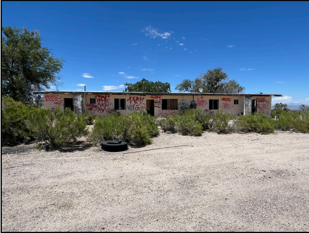
Plate 3.2–5: South façade of the residence, facing north.
