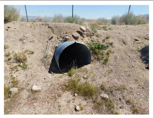
**Photograph 13:** A 36-inch culvert along the eastern boundary of the project site which directs flows from Drainage 5 to the northeast of the project site.
