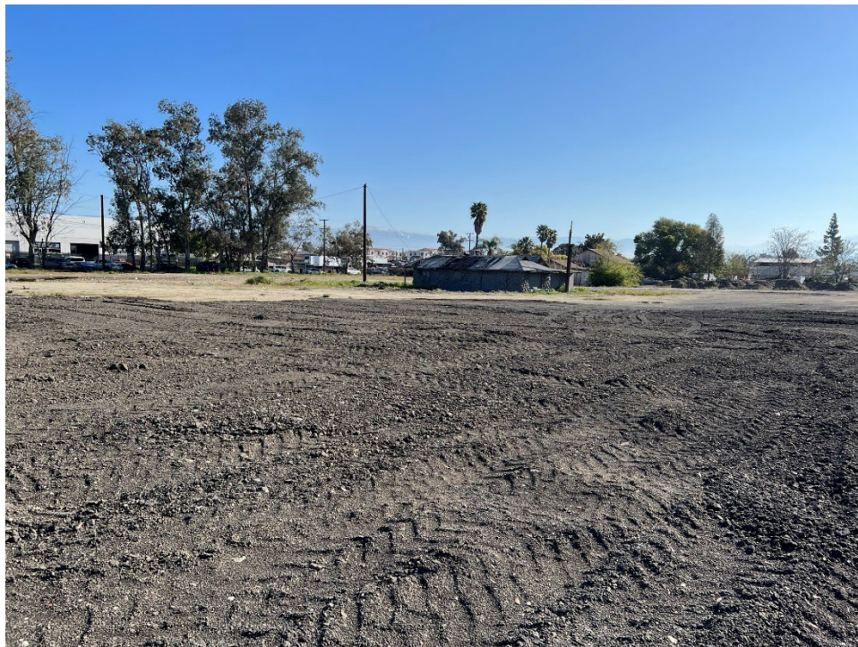
Photo 2 – Southwest corner of the Project site, facing northeast.
