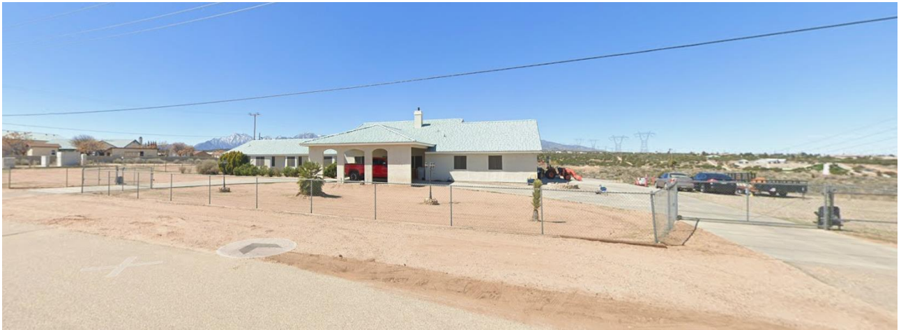
FIGURE 4: PROJECT SITE View looking southwest on Coriander Drive
