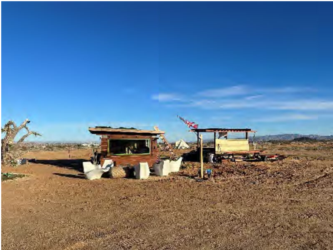
Photo 5: View of the existing structures near the northeast corner of the site.
