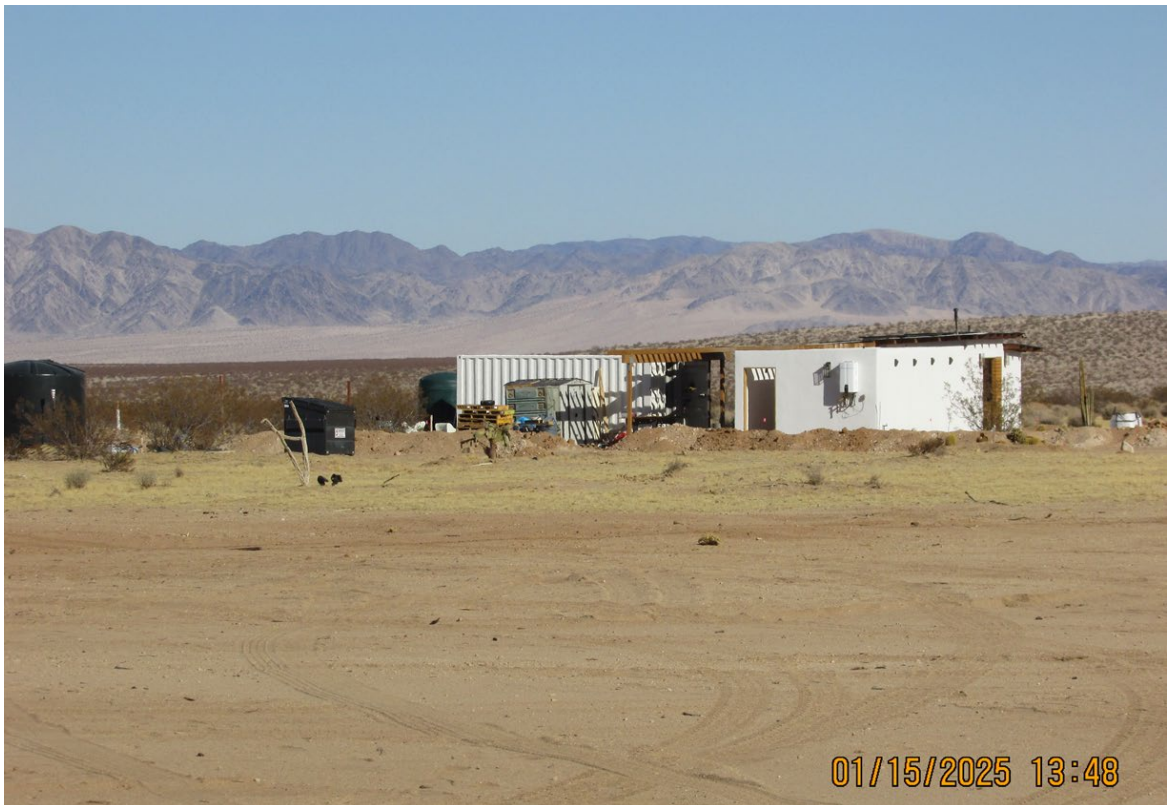
Photo 7: Exterior improvements of existing accessory structure.
