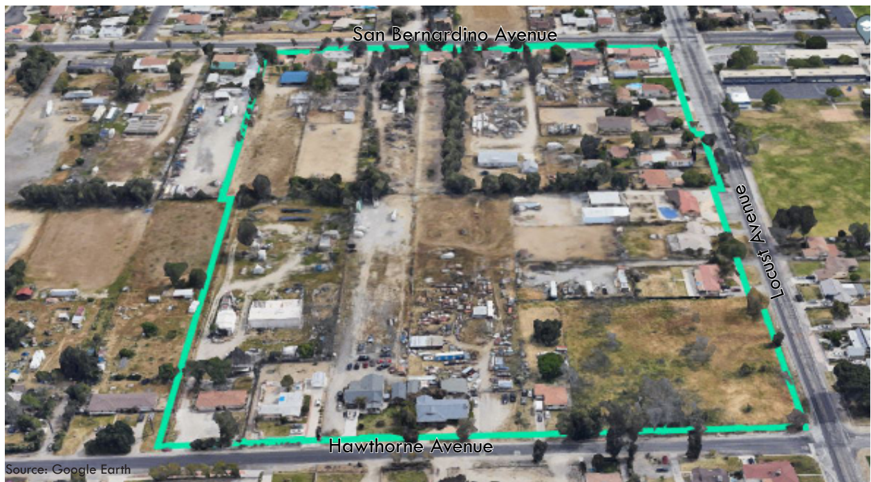
View looking south from the northern boundary of the Upzone site.
