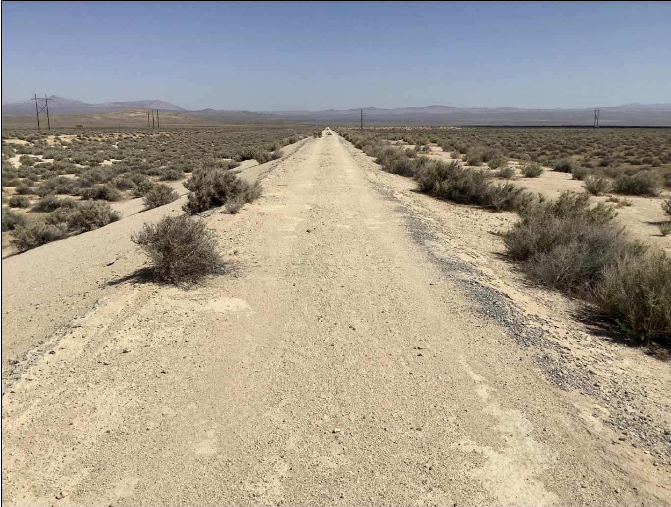
Figure 11. A levee runs north/ south along the western edge of the Original Survey Area, and diverts flow from an episodic dryland stream originating outside the property boundary.
